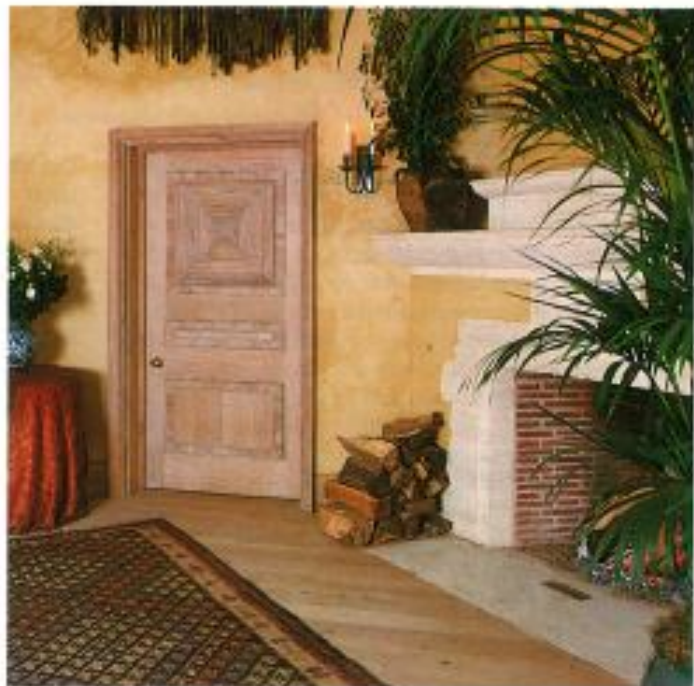
6—The chimneypiece in the principal room, and one of the limed oak doors, which have a square, reeded pattern
